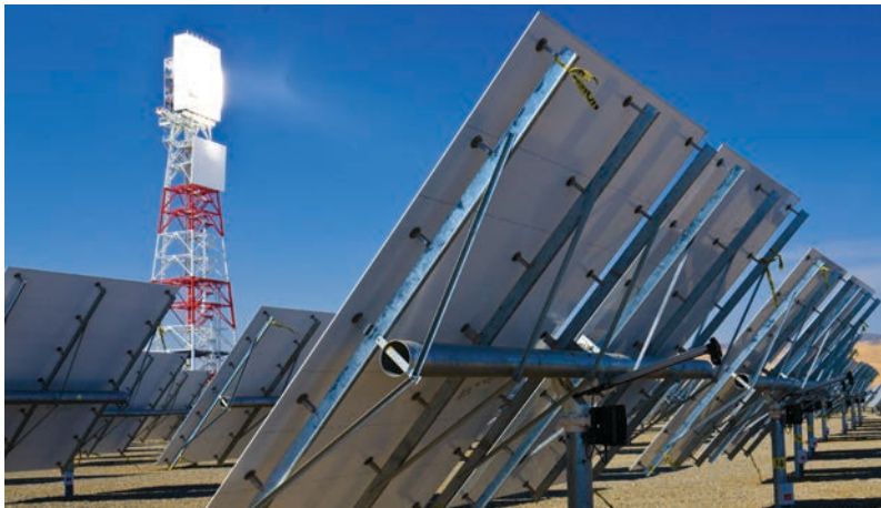
Solar Steam Generation Central Receiver, Coalinga, CA
