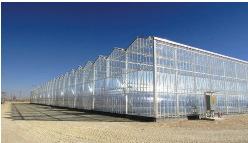
Solar Steam Generation Enclosed Trough, Amal, Oman
