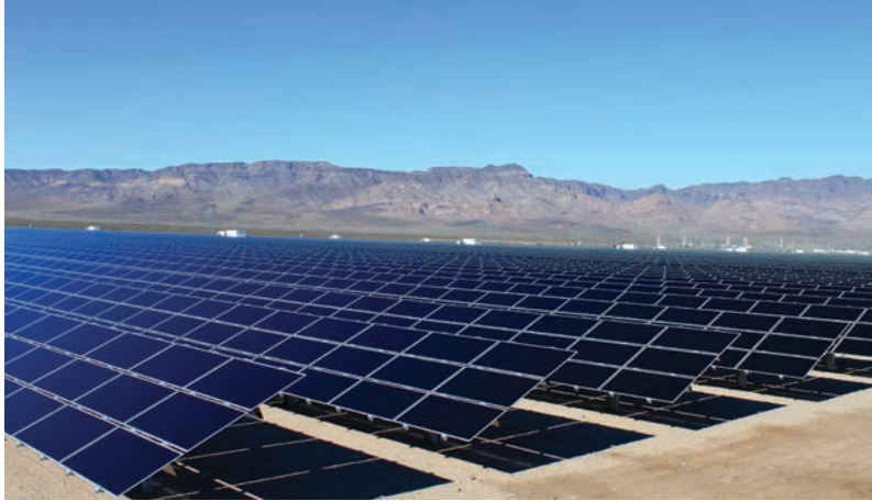
Solar Electric Power Generation
