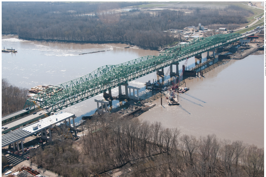
PHOTO: MISSOURI DEPARTMENT OF TRANSPORTATION, FLORENCE
